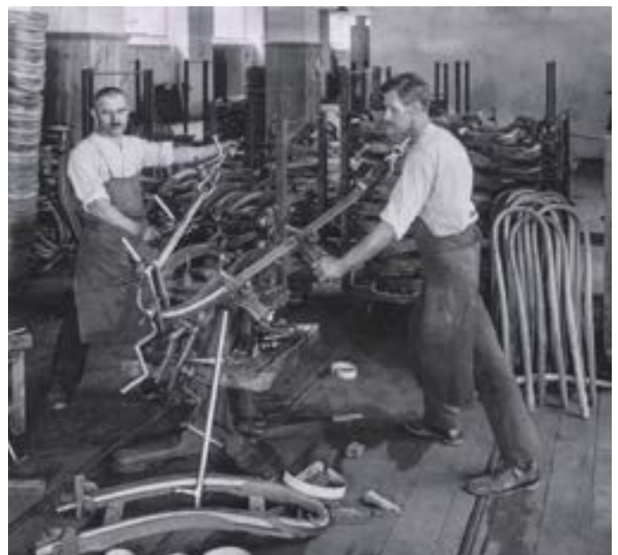
image: image of the bentwood process, 1929 [video showing Thonet's manufacturing methods]
